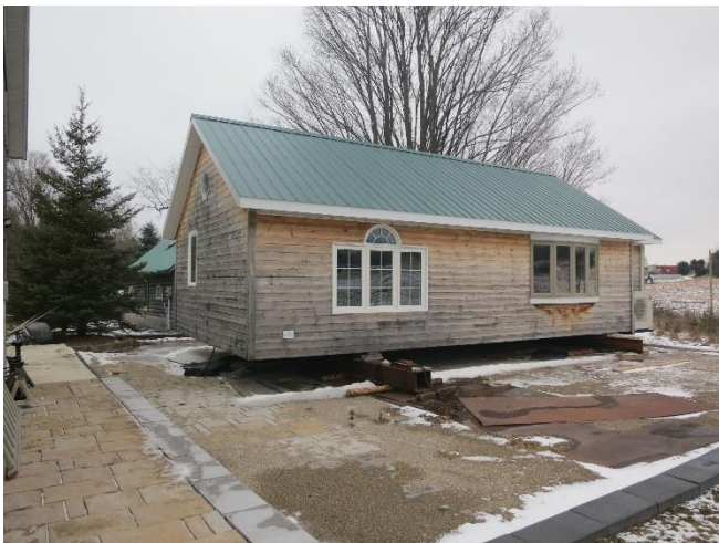
Photo 9: Existing accessory structure – proposed secondary dwelling unit – exterior view 3
