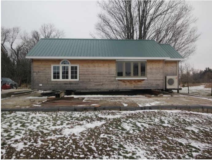
Photo 7: Existing accessory structure – proposed secondary dwelling unit – exterior view 1
