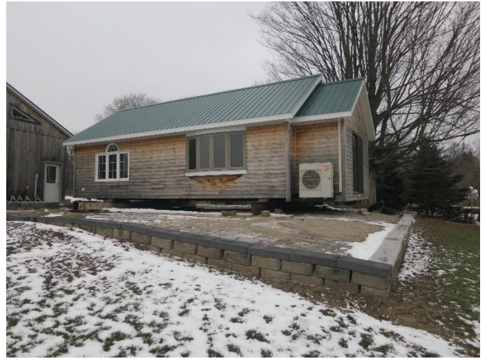
Photo 8: Existing accessory structure – proposed secondary dwelling unit – exterior view 2
