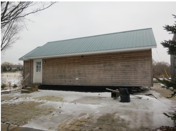
Photo 11: Existing accessory structure – proposed secondary dwelling unit – exterior view 5
