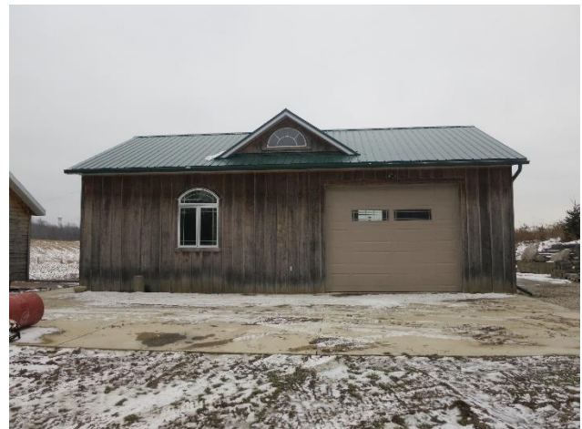
Photo 4: Workshop – accessory building – northwest cluster
