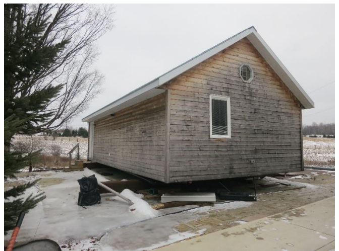
Photo 10: Existing accessory structure – proposed secondary dwelling unit – exterior view 4
