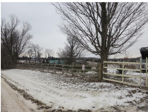
Photo 5: View of northwest cluster of accessory structures from Gold Creek Drive
