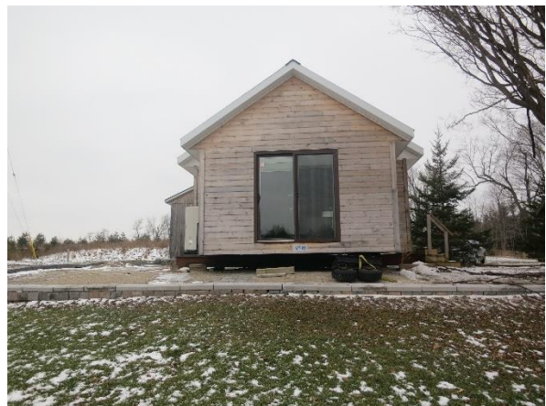
Photo 12: Existing accessory structure – proposed secondary dwelling unit – exterior view 6
