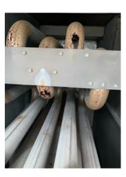
This unit can no longer function to provide heat to the main hall of the community centre. With the lead time of a new heat exchanger being 4-6 weeks, staff have ordered the replacement parts so that the unit will be functional prior to the heating season. The unit can still be used for cooling.
