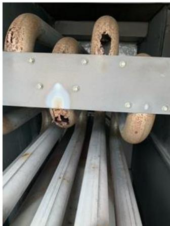
This unit can no longer function to provide heat to the main hall of the community centre. With the lead time of a new heat exchanger being 4-6 weeks, staff have ordered the replacement parts so that the unit will be functional prior to the heating season. The unit can still be used for cooling.
