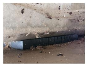
While no immediate structural concern exists, it is likely that there will continue to be premature deterioration of the girder ends if no action is taken. Replacement of the bearings and correction of the uneven loading of the bearings will increase the overall life of the superstructure.
