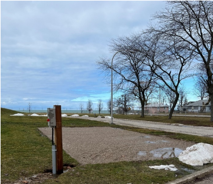
Figure 9: Gravel contractor trailer pad with a permanent electrical pedestal.
