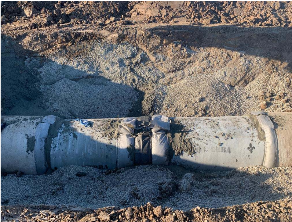
Figure 7: Completed pipe repair
