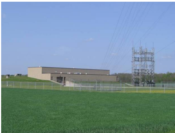
Figure 1: McGillivray Booster Pumping Station
