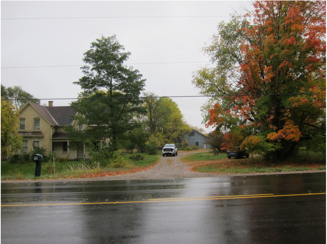
Photo No. 1. View of Subject Property main access (driveway) across from Gideon Drive looking southeast – former residential building is to the left.
