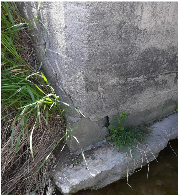
Wide Cracking of Abutment Face to Footing:
