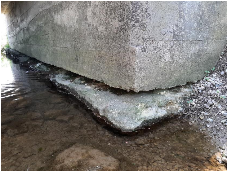
Wide Cracking of Abutment Face to Footing:
