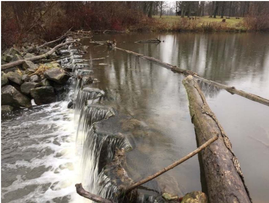
Photo 1: Coldstream dam constructed of vertical sheet piling and downstream armour stone.
