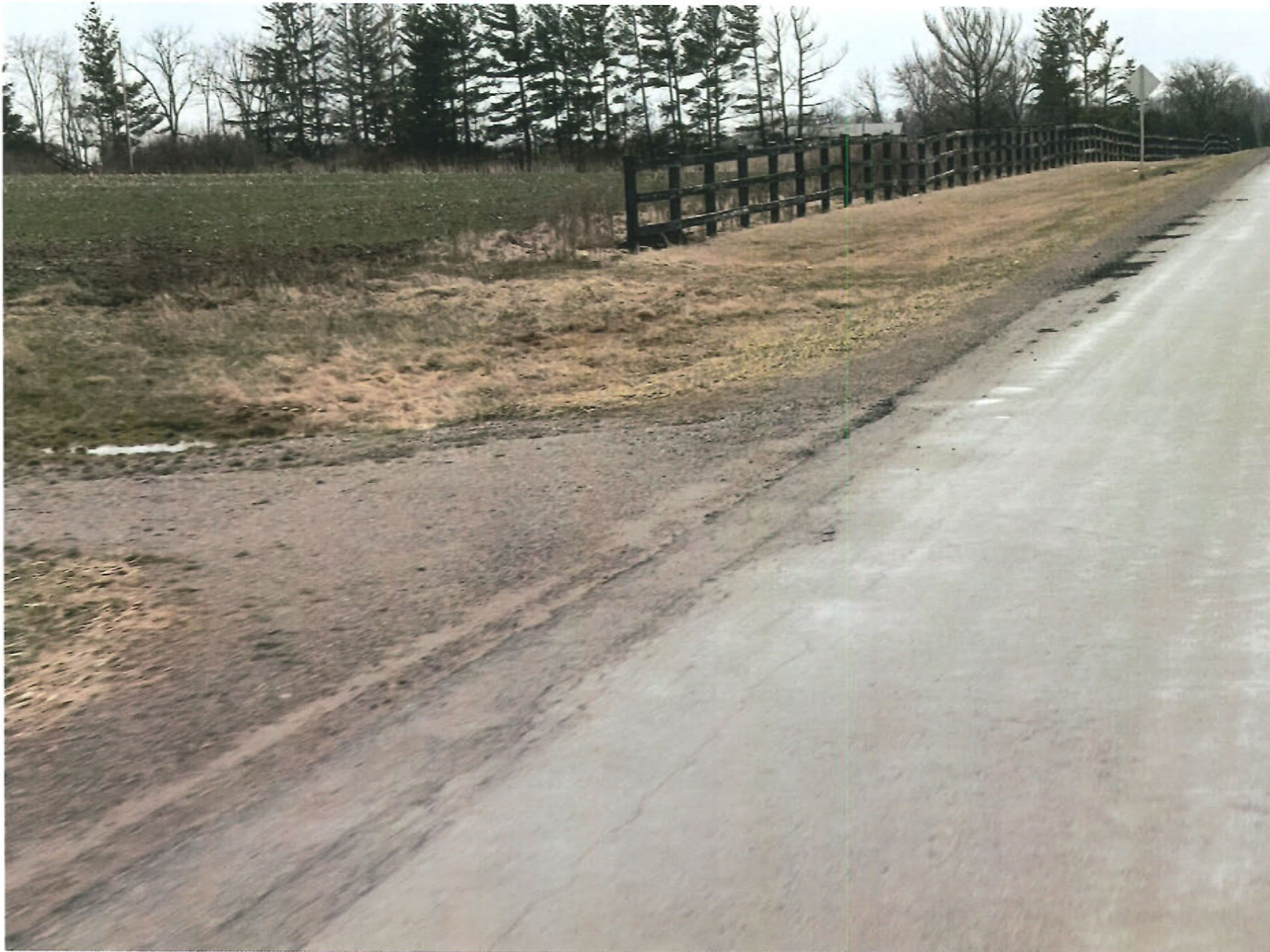
Figure 8 Suspected damage to municipal road near applicants' site, from applicants' vehicles using road during half load season with axle weights >5,000kg.
