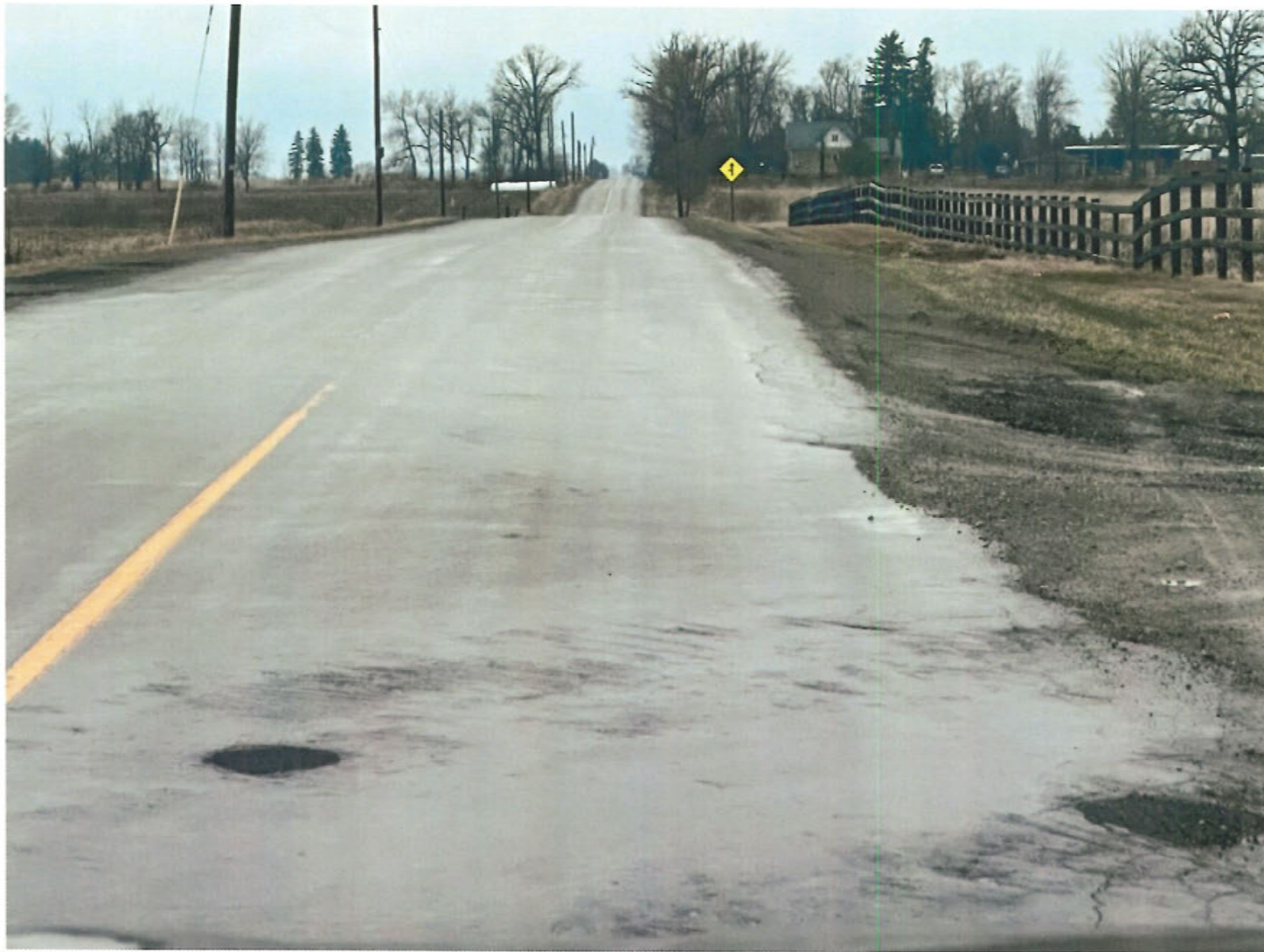
Figure 6 Damage to municipal road from applications excavator tracking on road to property on cook and decker drive.
