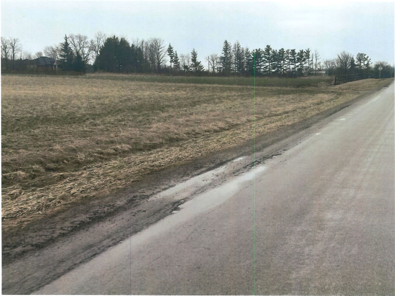
Figure 7 Suspected damage to road from applicants' vehicles using road during half load season with axle weights >5,000kg.
