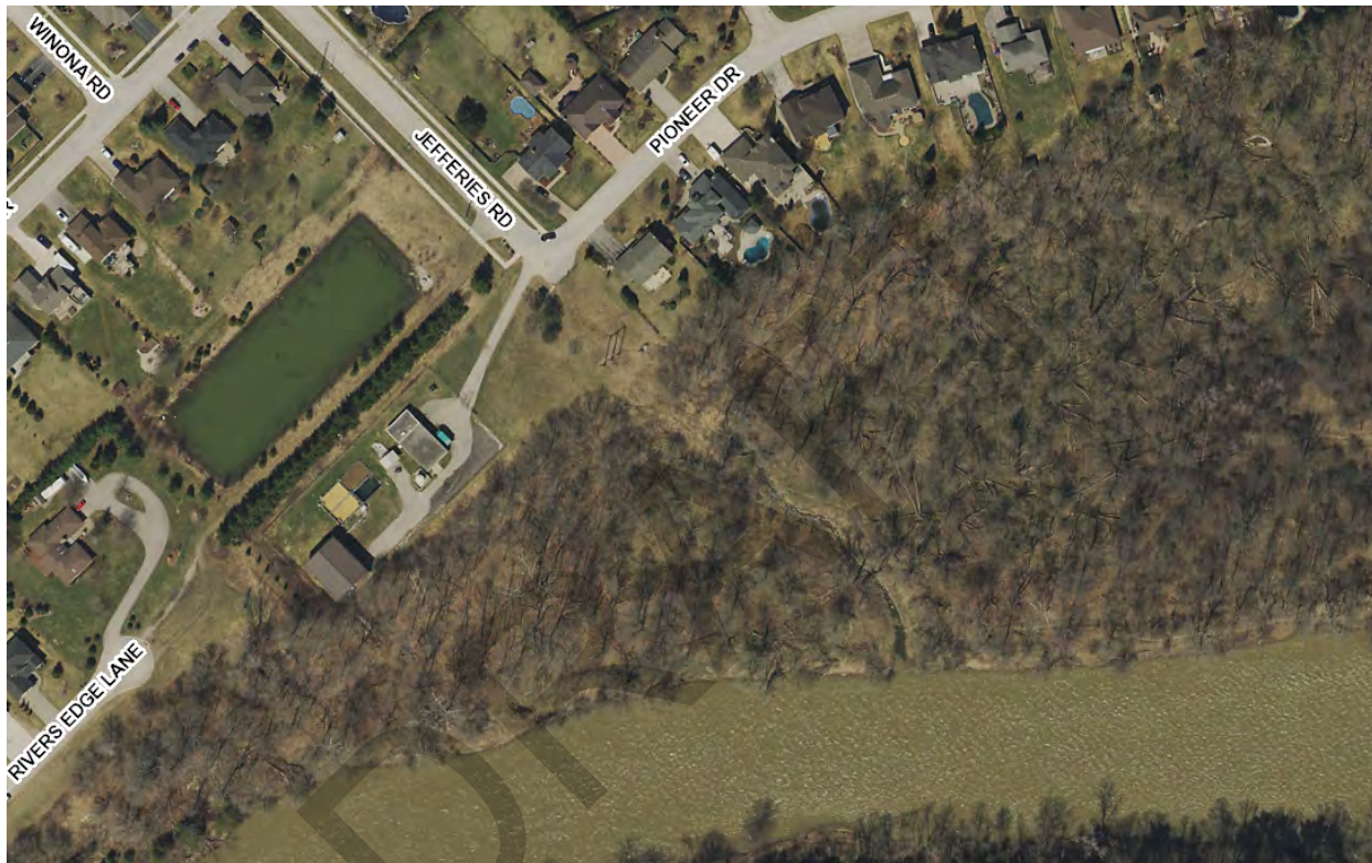
Figure 2: Jefferies Road Pump Station and Thames Riverbank
