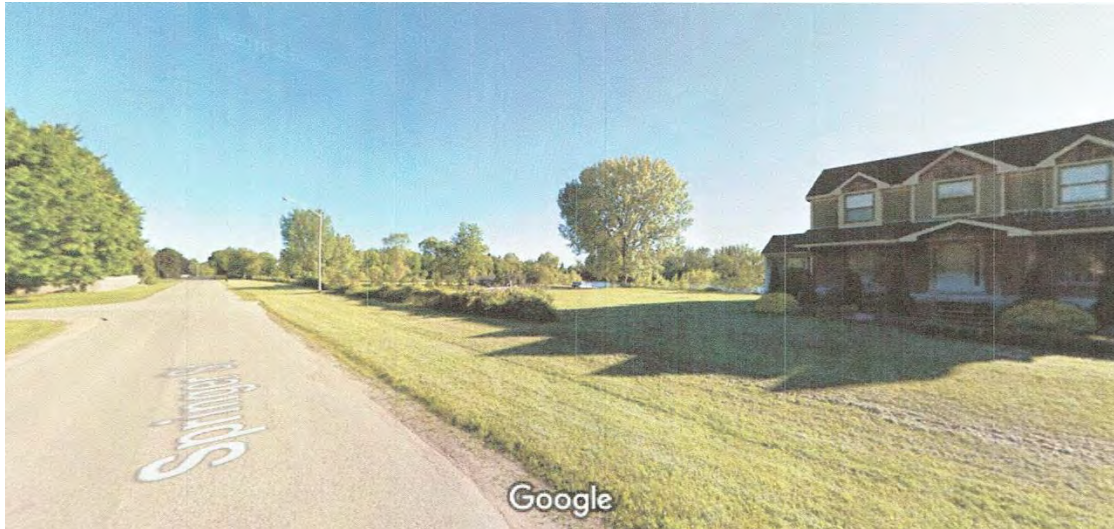
Figure 3: Street view - Subject Lands – Springer Street Frontage showing Snyder residence at 45 Springer Street and then the location of the 8 proposed single detached lots with the owners existing large residence that would be made into a semi-detached residence. (Source: Google Maps, 2014)
